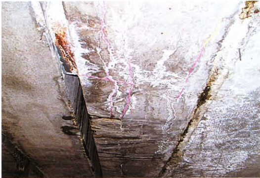
PC桁のひび割れ・遊離石灰
