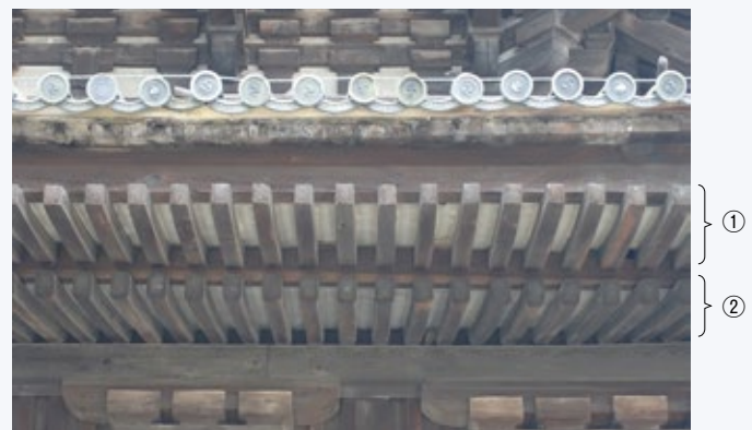
Kohfuku-ji Temple five-storey pagoda rafters (Courtesy of Kohfuku-ji)
