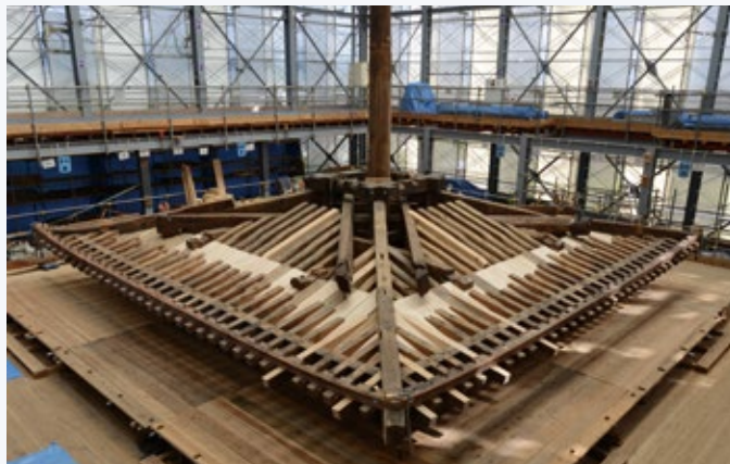
Yakushi-ji Temple's East Pagoda disassembly and repairs (Courtesy of Yakushi-ji)
